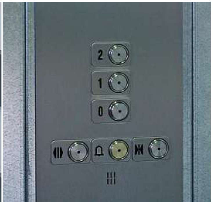
Car control panel of stainless steel, vandal-proof
