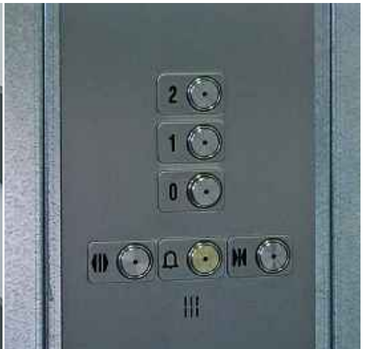
Car control panel of stainless steel, vandal-proof
