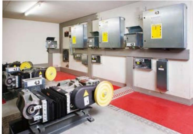
Triplex commercial installation powered by DR SGB 142 linked with a CO MX control
