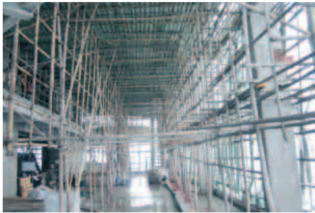
Photo below, top: Rigging used for applying interior finishes. Photo credit: Guido Gilli, Jardine Schindler Hong Kong. Photo below, middle: Technicians install the newest generation of Schindler high-performance elevator drives. Photo credit: Hanspeter Köpfl, Andreas Ryser, Jardine Schindler Hong Kong. Photo below, bottom: The International Commerce Centre rises to become part of Hong Kong's skyline. Photo credit: Sun Hung Kai Properties.
