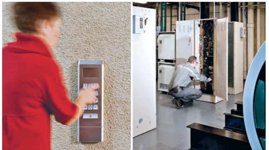
Photo left: A visitor accesses a Schindler ID terminal. Photo right: A technician inspects the new Schindler ID controllers in the machine room. With the controllers, fixtures and cars all upgraded, 680 N. Lake Shore Drive has the most efficient elevator system in its long history.
