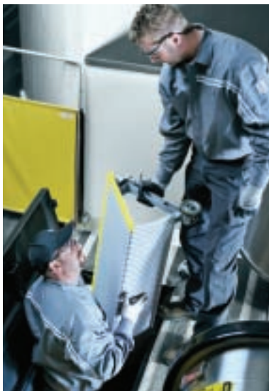
Photo above: Schindler technicians install new steps as part of an escalator upgrade. Photo right: Fully upgraded escalators can look and perform like new at lower cost and with less inconvenience.
