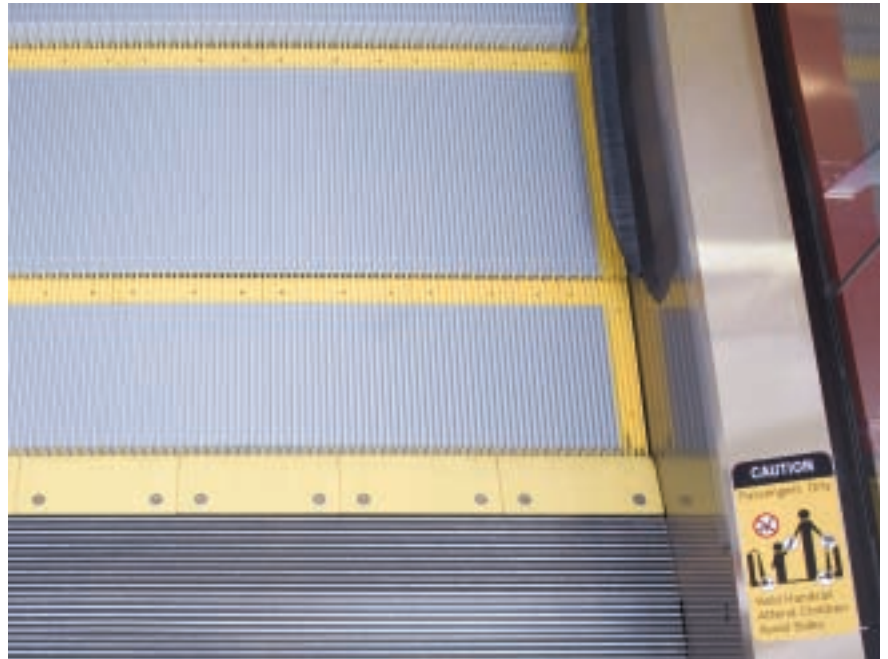
Photo above: Bright yellow safety and step guides keep passengers alert while entering and exiting the escalator. Skirt deflector brushes help prevent skirt panel entrapments and Hold Handrail signs announce ridership rules. Photo left: Schindler technicians run upgraded escalators through a full range of performance tests to ensure they meet all performance parameters.
