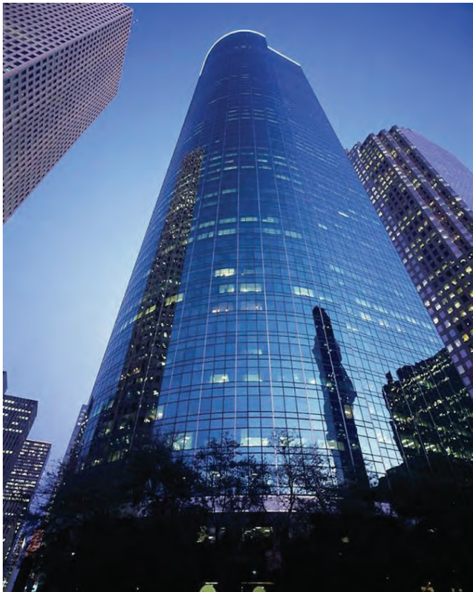
▶ Houston's Wells Fargo Plaza, built in 1982, is getting a new elevator system, including 11 double-deck Schindler units; photo courtesy of Wells Fargo Plaza.
