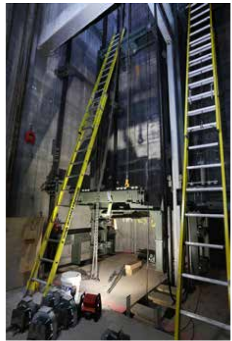
Installing the service car frame and platform
