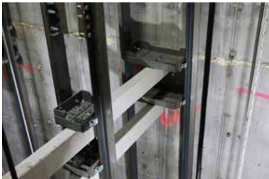
Rail brackets and rails with a double divider to meet seismic rail-spacing requirements
