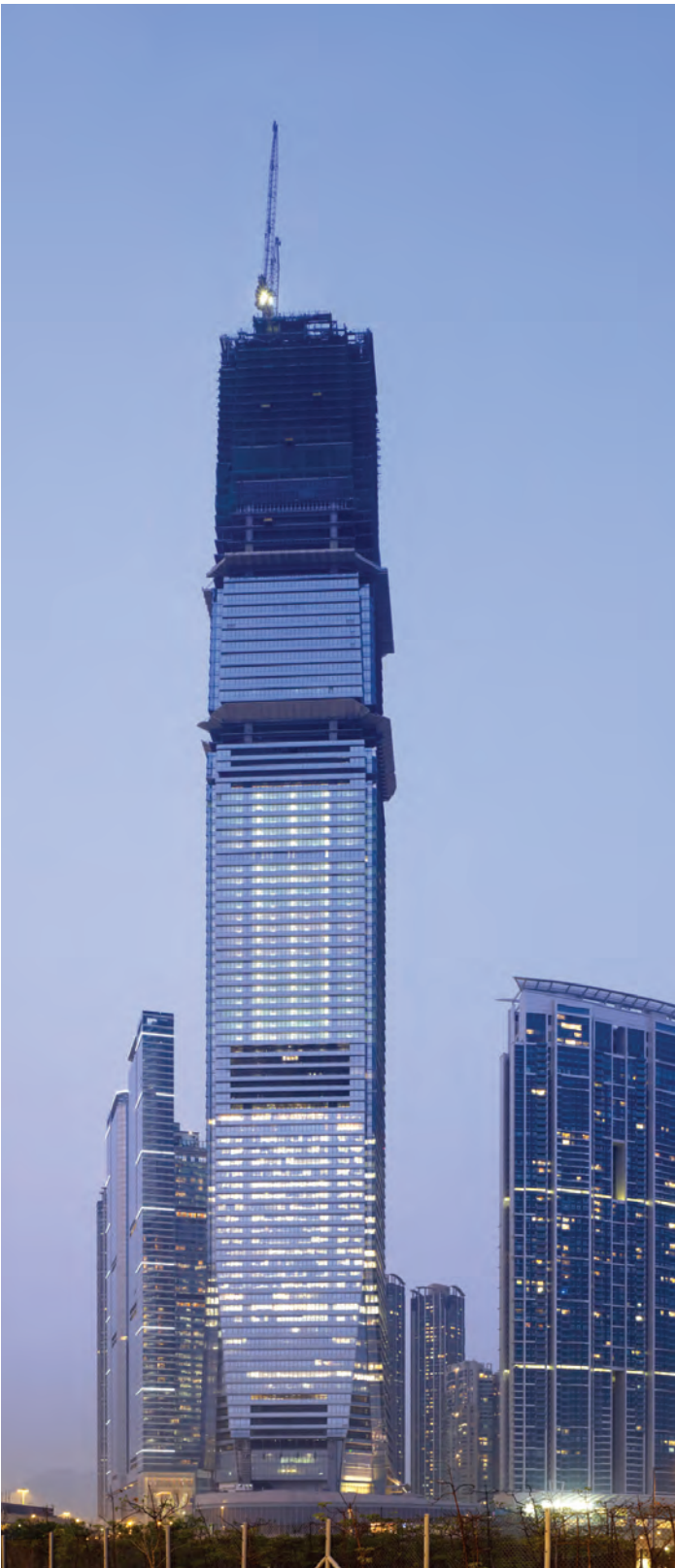
Figure 3: The tower under construction
