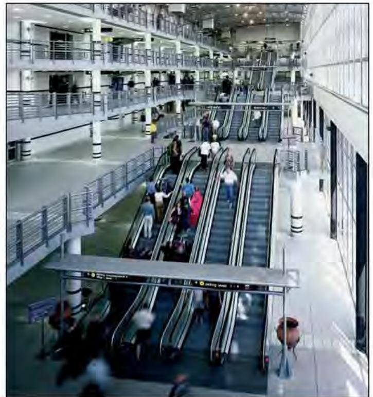
*Taking a lifecycle approach to escalators, a properly designed and maintained truss and framework typically should have an indefinite life. Partnering and consulting early in the design process with manufacturers can help yield potential savings through optimal configurations.*
