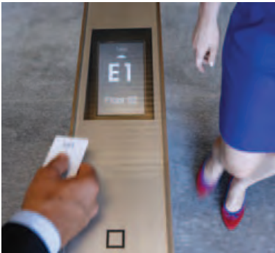
Photo above: Card readers are incorporated into turnstiles to offer tenants personalized service to bring them to their destination floor. Photo below, right: Black granite lobby walls provide a dramatic foreground for the polished African hardwood that leads to the elevator banks.
