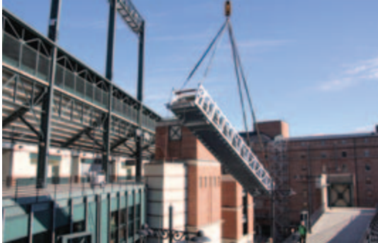
Photos, page 30: A crane lifts the Schindler 9700 over the Oriole Stadium wall. Photo credits: Phil Cohen, Maryland Stadium Authority.
