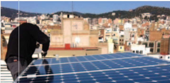
The Schindler Solar Elevator replaces the use of net energy by using solar panels.
