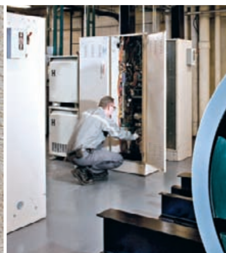
Photo left: A visitor accesses a Schindler ID terminal. Photo right: A technician inspects the new Schindler ID controllers in the machine room. With the controllers, fixtures and cars all upgraded, 680 N. Lake Shore Drive has the most efficient elevator system in its long history.
