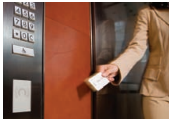
Schindler ID® destination-dispatch system with access control is gaining widespread use for enhanced building security. Passengers identify themselves with a badge, PIN code or other electronically readable device. The system automatically assigns an elevator car that conforms to their approved level of access.
