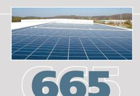
The 665 kilowatt photovoltaic solar array at Hanover generates half of the building's total annual power consumption and provides renewable energy year-round.
