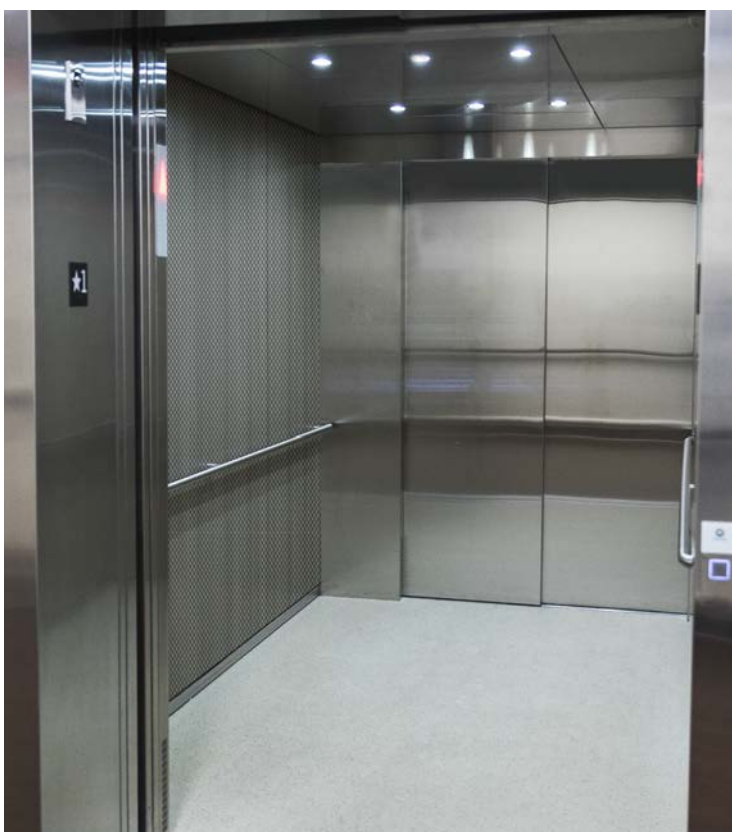
5WL Stainless Steel wall finish Finish: 5WL Stainless Steel Handrails: Round handrails on side walls Ceiling: Brushed stainless steel with spot lighting
