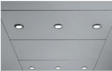
Ceiling lighting - standard LED round spot downlights*
