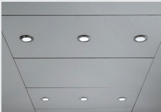
Ceiling lighting - standard LED round spot downlights**
