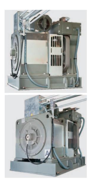
Schindler modular gearless machines are specifically designed to simplify installation in existing machine rooms, while maintaining optimised ride quality. They can be disassembled at the job site and then reassembled in the machine room.
