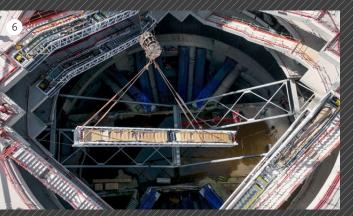
A crane lowers the escalators into the shaft, assisted by lifting straps.
