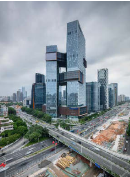
The building with towers that are angled towards each other – connected by the two recovery decks
