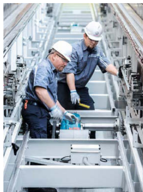
Modernization of an escalator using 'InTruss'
