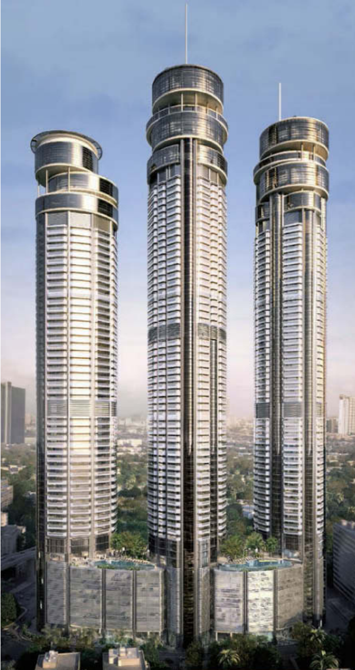
Omkar Worli 1973, residential buildings; Mumbai, India
