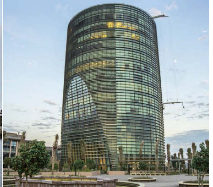
Alturki Business Park, office building; Al Khobar, Saudi Arabia
