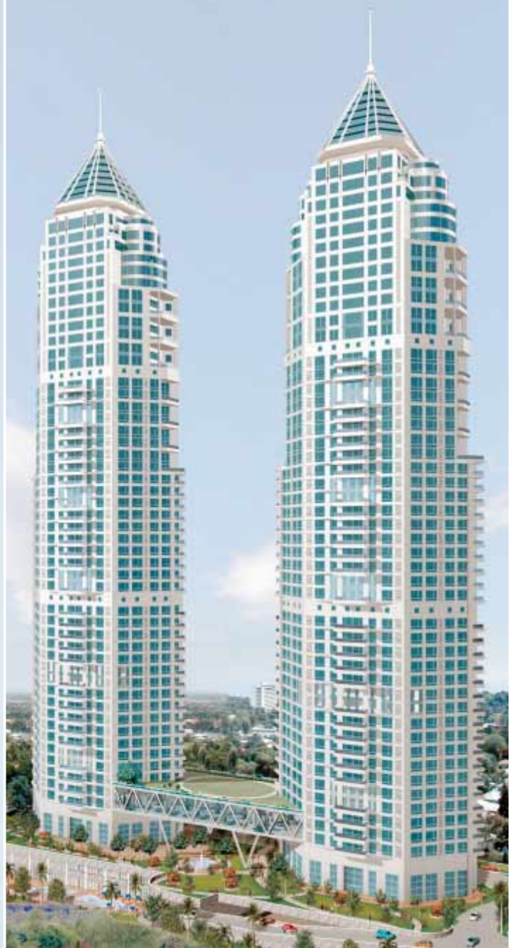
Imperial Towers; Mumbai, India
