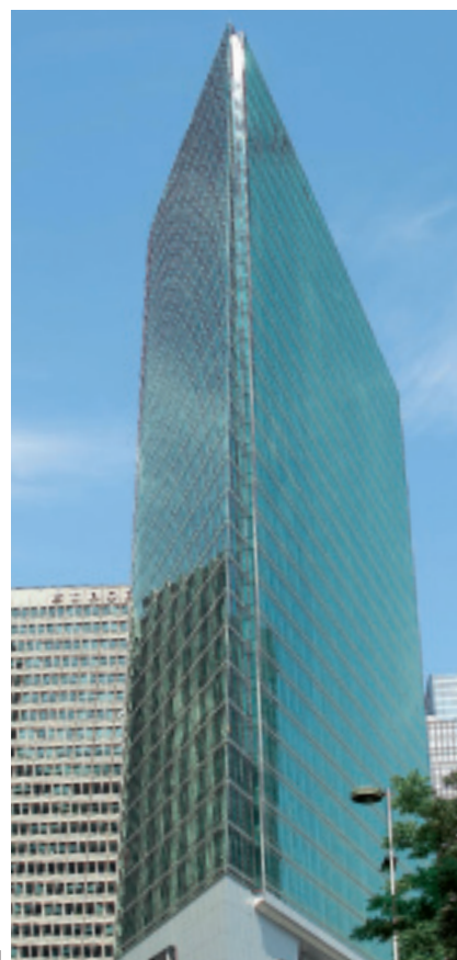
1 CBX Tower: 10 Schindler 700 high-rise elevators equipped with the Miconic 10 hall call destination control system and Schindler/D access control system, plus three further elevators; Paris, France
