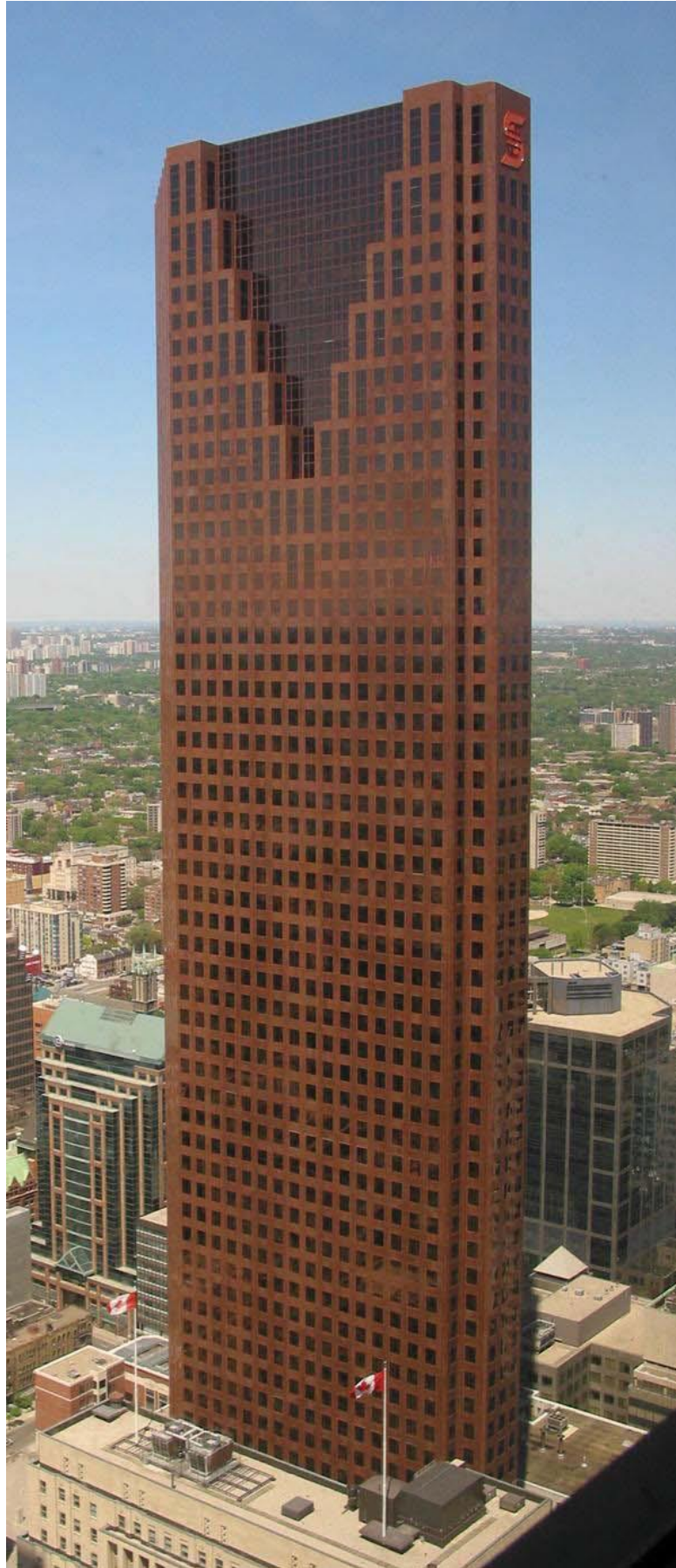
Modernization of Scotia Plaza, Toronto, Canada
