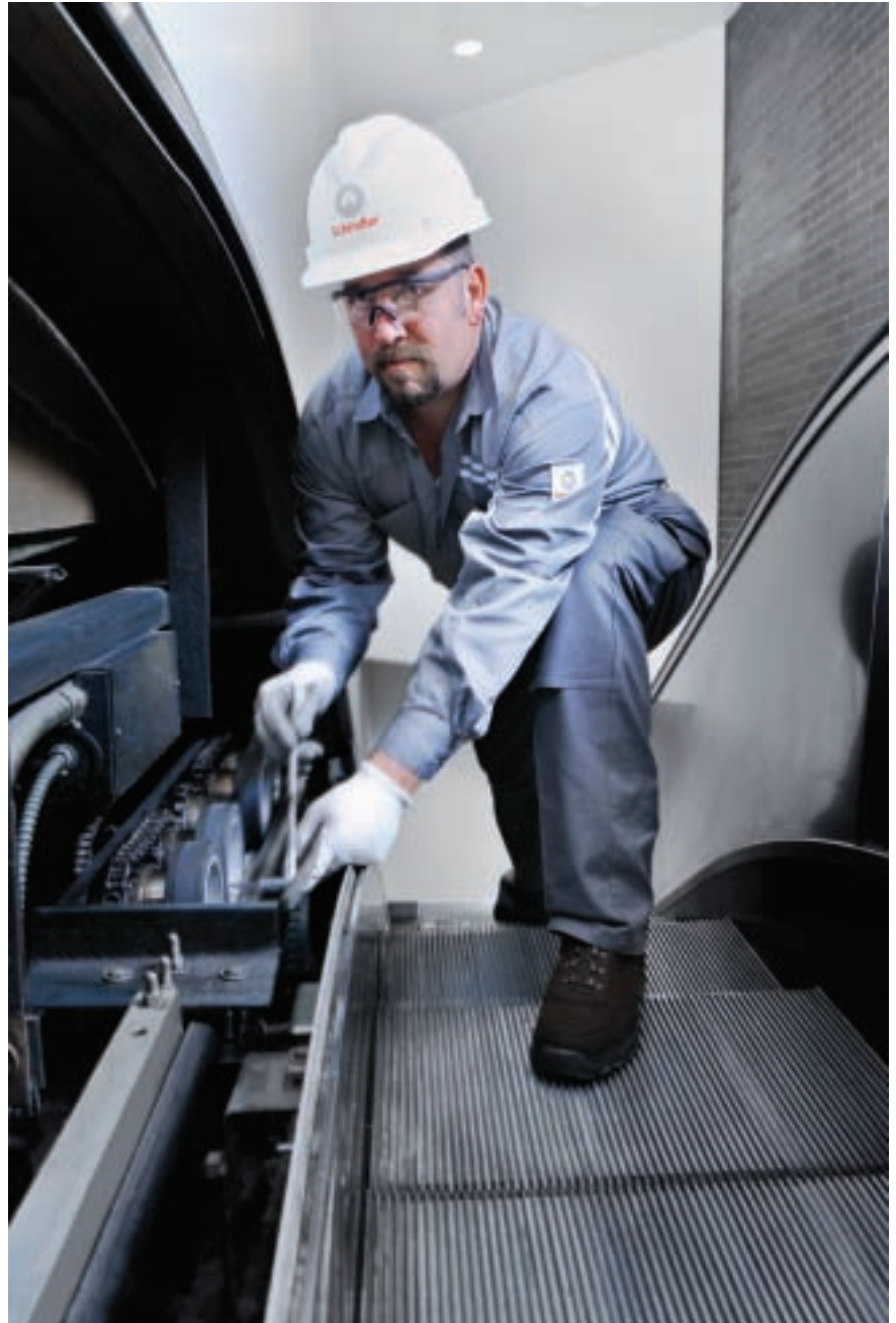
Schindler technician makes precision adjustments to new handrail drive assembly.
