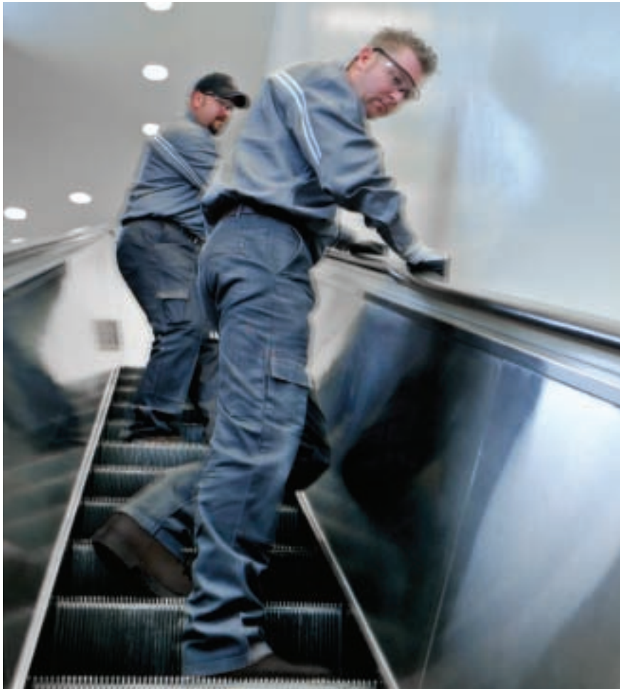
Photo above: Schindler technicians remove old handrail. Photo right: The new handrail drive assembly. Photo far right: The new handrail speed monitor.
