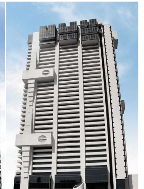
ABSA Tower, Pretoria, South Africa
