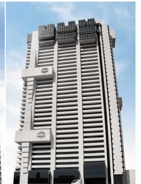
ABSA Tower, Pretoria, South Africa
